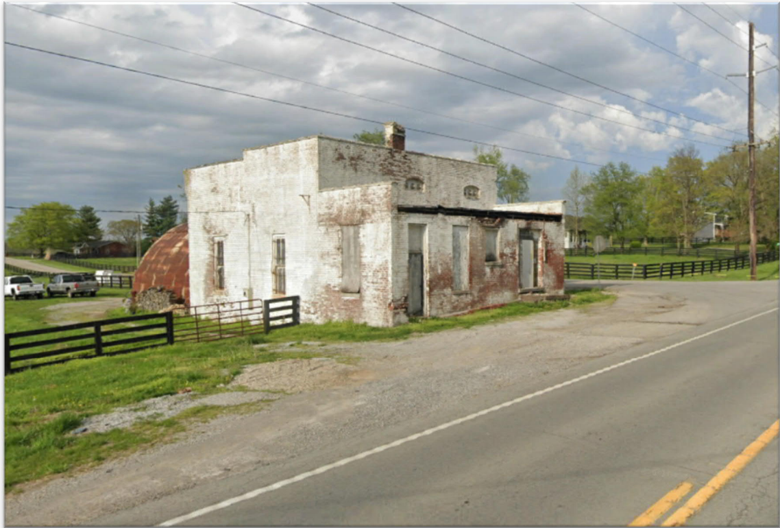
Plate 2: Looking east toward Scott Station Power House
