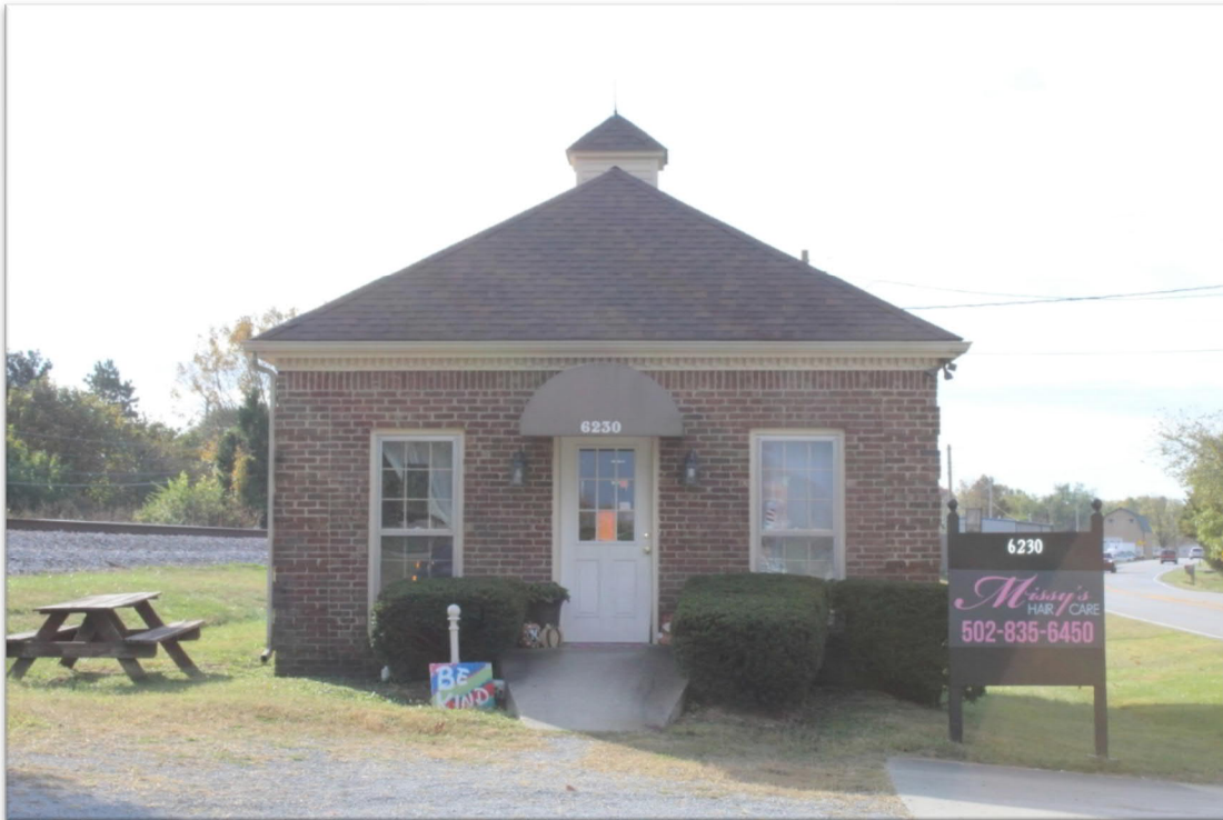
Plate 4: Looking south toward Camden Station/Missy's Hair Care
