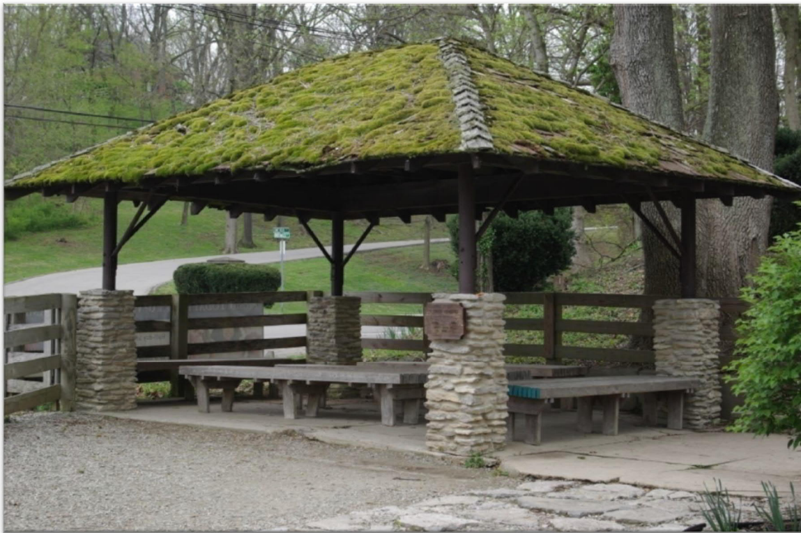
Plate 11: Looking southeast toward the Florida Heights Station
