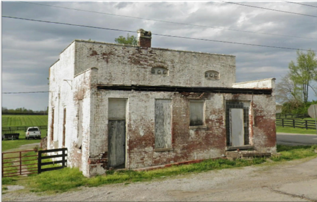
Plate 1: Looking northeast toward the Scott Station Power House
